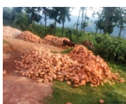
New Church Construction
